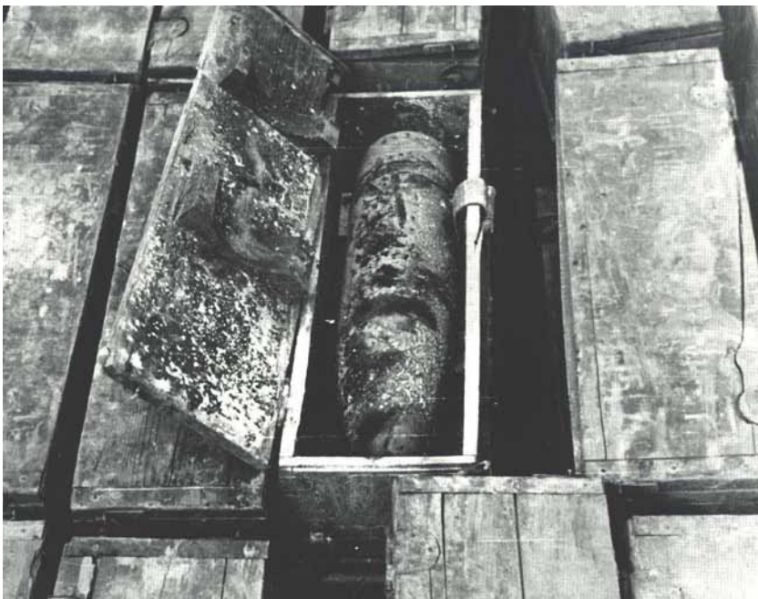
Figure 20: Leaking chemical munitions were sometimes encountered during the trafficking of chemical warfare materials for sea-dumping. This item, leaking sulfur mustard, was encountered during handling in Bremerhaven under control of the U.S. Military Administration in Germany. It was reported to have been decontaminated later. Another general option to cope with such dangerous items was emergency sea-dumping (HELCOM 2011c).
