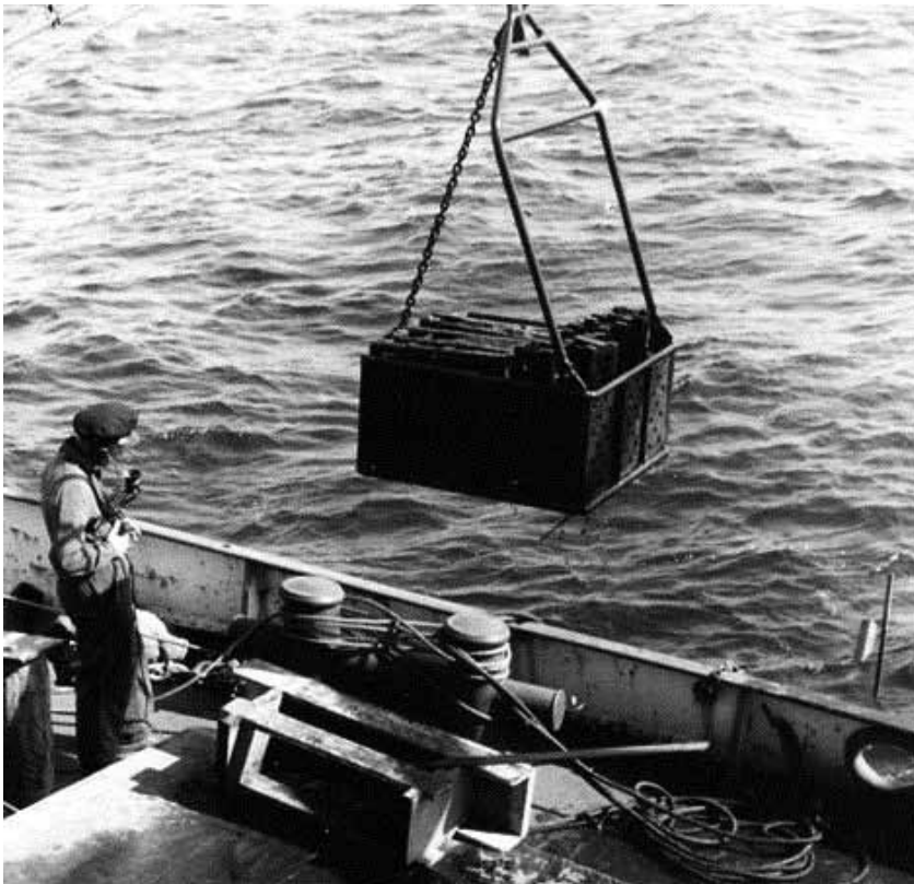
Figure 21: A basket filled with 10.5 cm Tabun shells is heaved on board from the wreck of the 1,000 tonnes barge in 1959/1960, which had been scuttled on behalf of the Germany Navy before the end of the war in 1945 (Kinder 1960).
